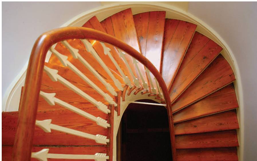
The staircase features arrow-shaped balusters.
